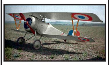
that were to perform most air combat duties for the rest of the war. It would seem most natural to place the gun between the pilot and the propeller, firing in the direct machine guns were prone. However, this presented an obvious problem: a percentage of bullets fired "free" through a revolving propeller will strike the blades, with predictable results.
